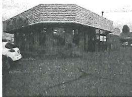
2 - VIEW OF SOUTH EAST SIDE
