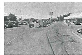
6 - VIEW OF PARKING LOT LOOKING WEST
